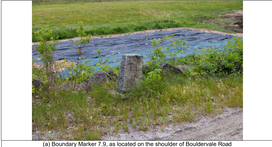
(a) Boundary Marker 7.9, as located on the shoulder of Bouldervale Road
